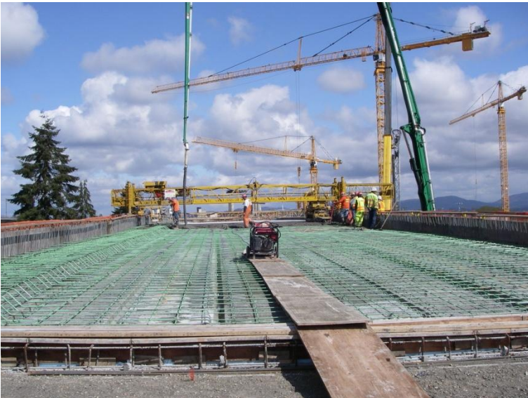
Bridge #4 Concrete Placement
