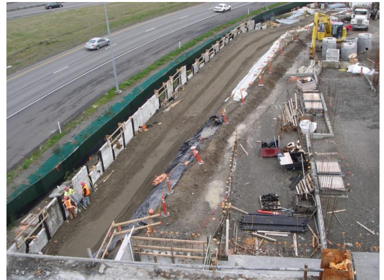
MSE Wall #1 Installation Progress
