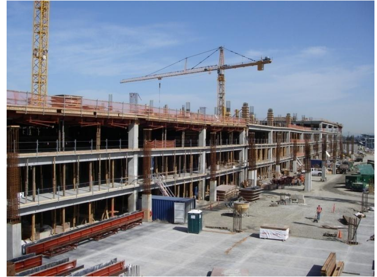
Elevated Decks in Areas A, B and C
