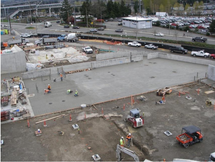
QTA #1 Slab-on-Grade Placement
